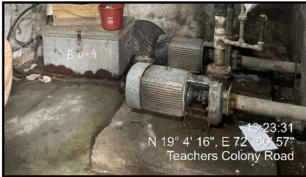
most efficient pump
