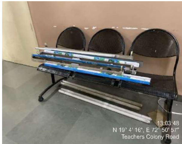
Replacing with led lights
