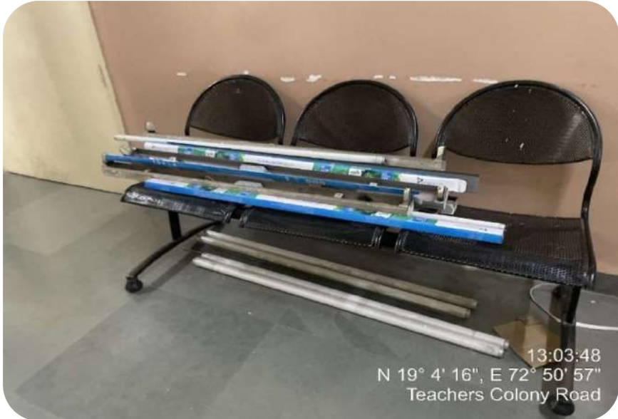
Replacement of LED lights with old one
