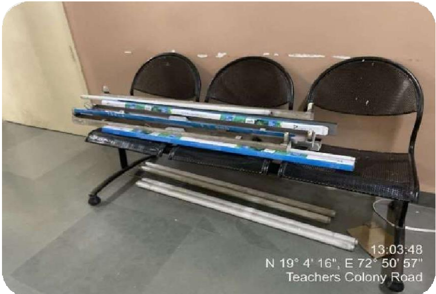
Replacement of LED lights with old one
