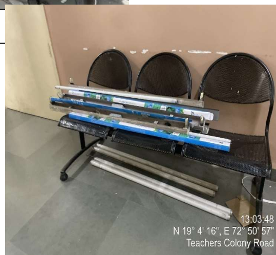
Replacing with led lights
